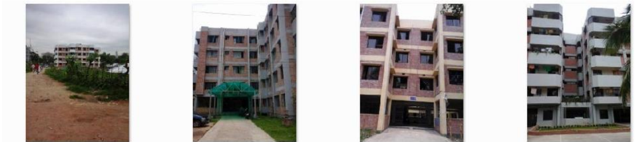
Plate 1. Residential buildings of SAU
