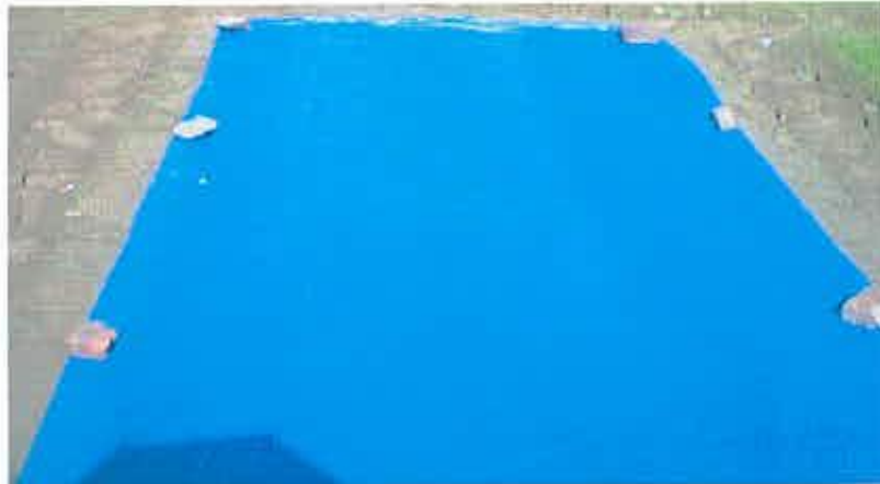
Plate 3 a. Placing polythene for bed preparation
